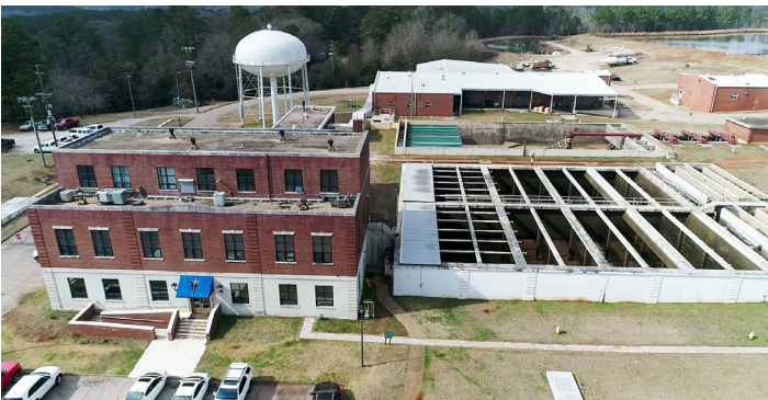
Walter Williams Filtration Plant
