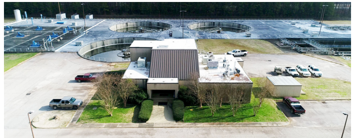
Long Cane Wastewater Treatment Plant
