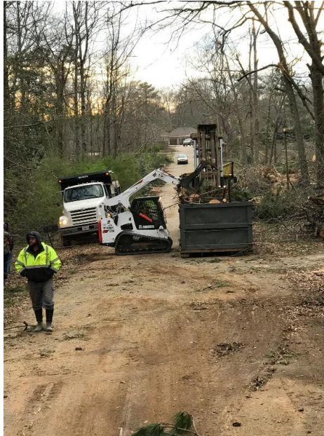
Public Works crews clearing storm debris in Pine Mountain
